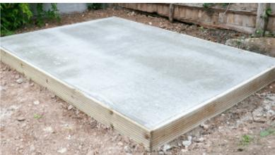
Remove any vegetation from the area. Pour the concrete approximately 2" deep using 5:1 ballast to cement mix. Suitable for all bases if sufficient foundation ballast installed.
