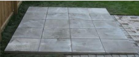
Remove any vegetation from the area and lay the slabs onto sand or ballast. Ensure using a spirit level that the slabs are level. A suitable base for all buildings is sufficient foundation ballast installed.
